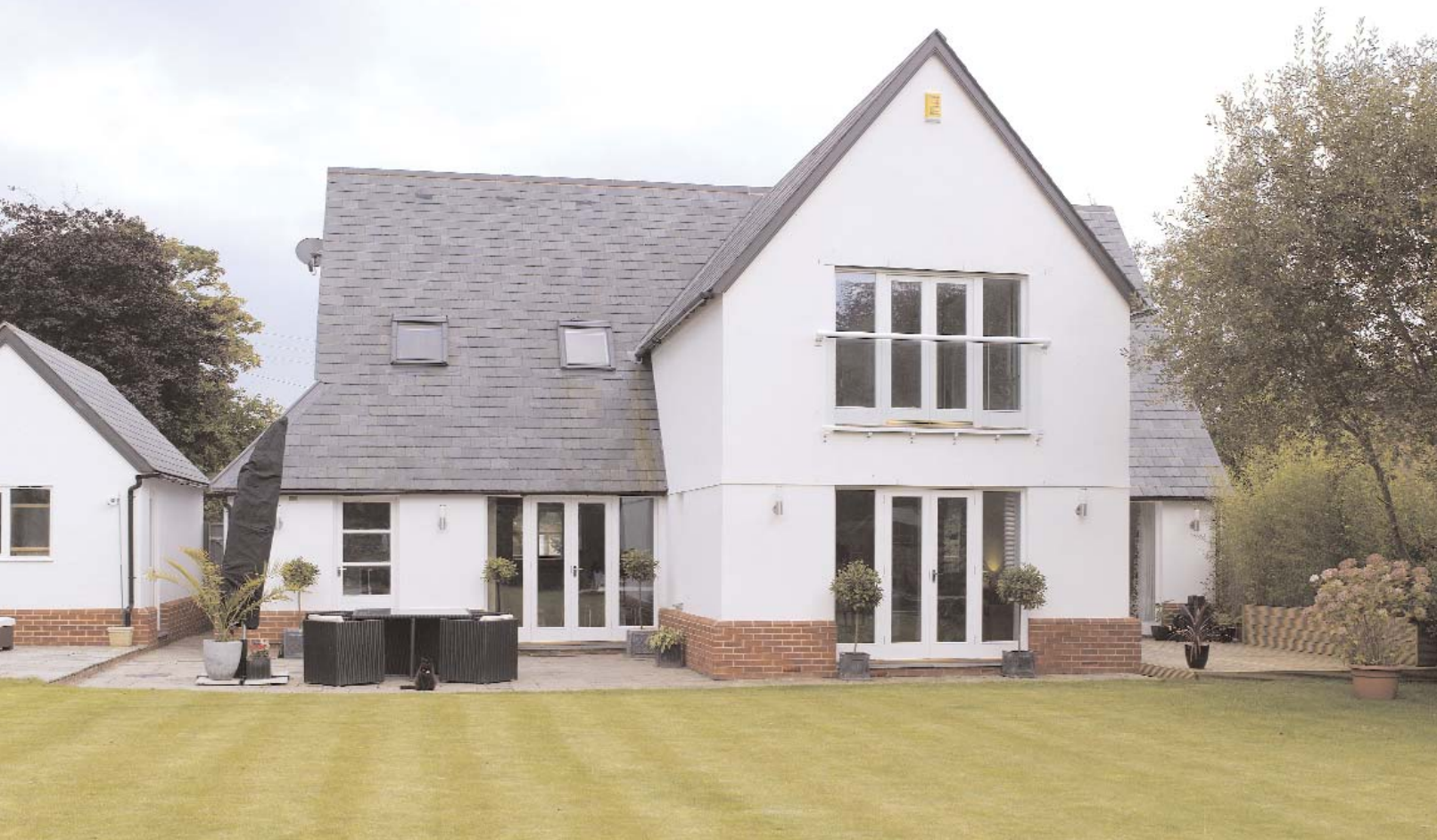
ABOVE: Four sets of French doors open the house out to the rear, with a balcony leading out from the master bedroom; the rooflights are an effective way to introduce extra light into the rear of the first floor, where the ridge height was affected by planning restrictions
